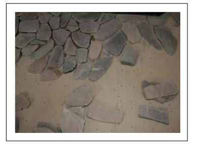
In most cases, it will be necessary to trim the stone edges in order to make clean transitions to adjacent floors. The easiest way to make a clean line next to a wall or a dividing floor is to trim an edge on the Thin Veneer. We recommend that the stone is trimmed and set 1/4" from the floor adjacent to it. Then fill the 1/4" space with flexible caulking prior to grouting which will accommodate movement from the adjoining floor.
